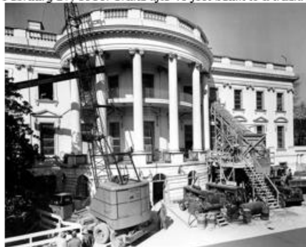
February 27, 1950: Crane lifts 40-foot beam to a truck.
