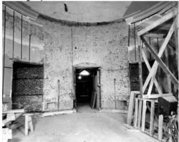
February 23, 1950: Workers remove the main staircase
